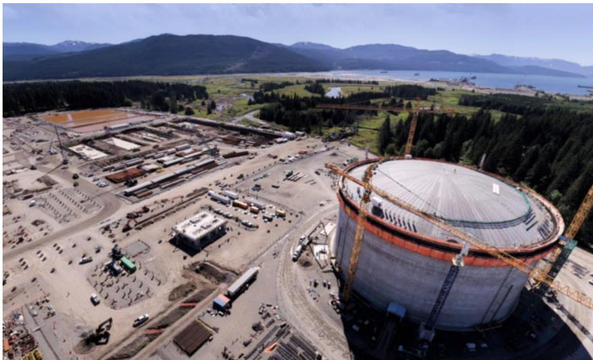
**Figure 4 LNG Storage Tank (2021 Q3)**
