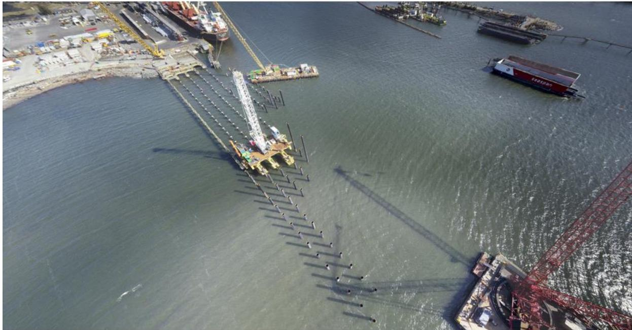
**Figure 1** Terminal A construction – piling for foundation
