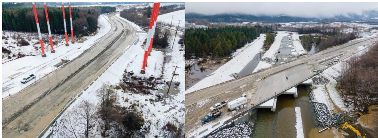
Figure 3-1 Moore Creek & Anderson Creek Bridges (Q4 2020)
