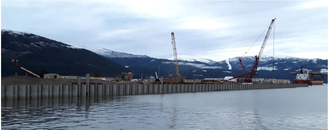
Figure 3-4 Quay Wall at the Berth (Q4 2020)
