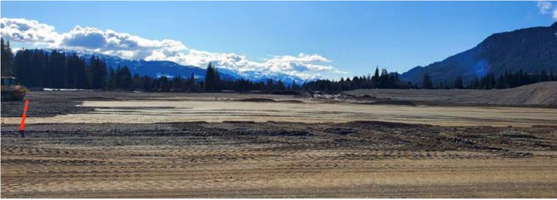
PHOTO 1: SITE PREPARATION ACTIVITIES (MARCH 2020)
