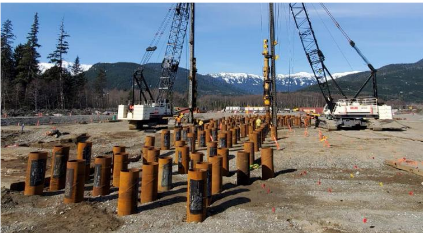
PHOTO 6: RIGID INCLUSIONS FOR GROUND IMPROVEMENT AT LNG STORAGE TANK SITE (MARCH 2020)
