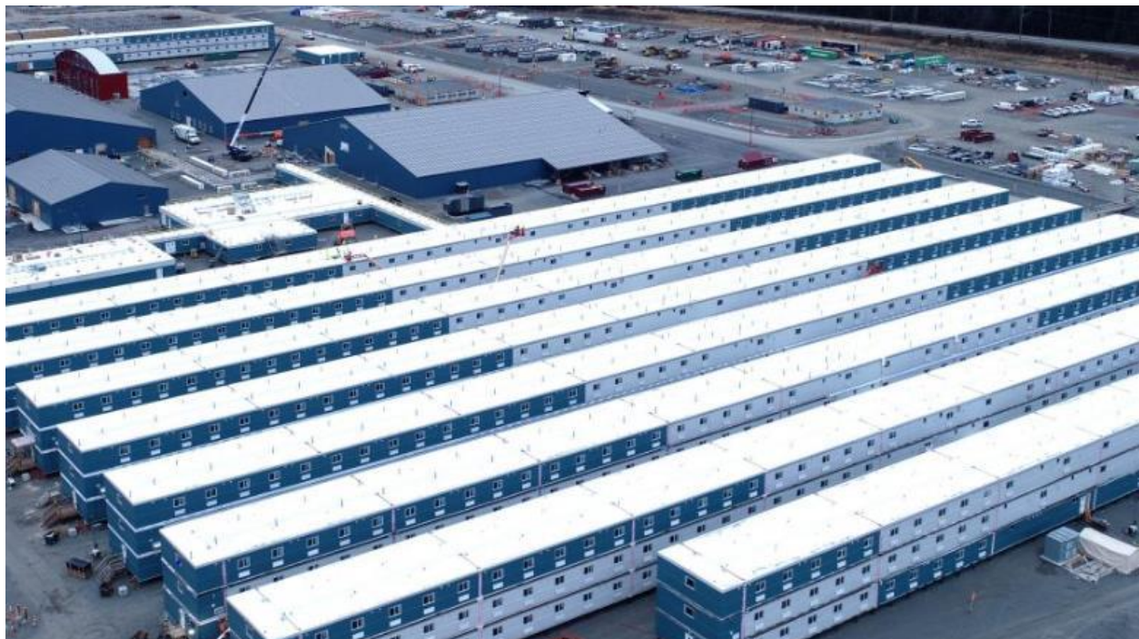
Figure 2 Cedar Valley Lodge Under Construction (December 2019)
