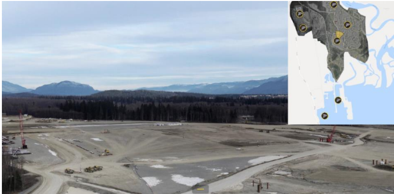
Figure 1 Site Preparation of LNG Train Area facing Northwest (December 2019)
