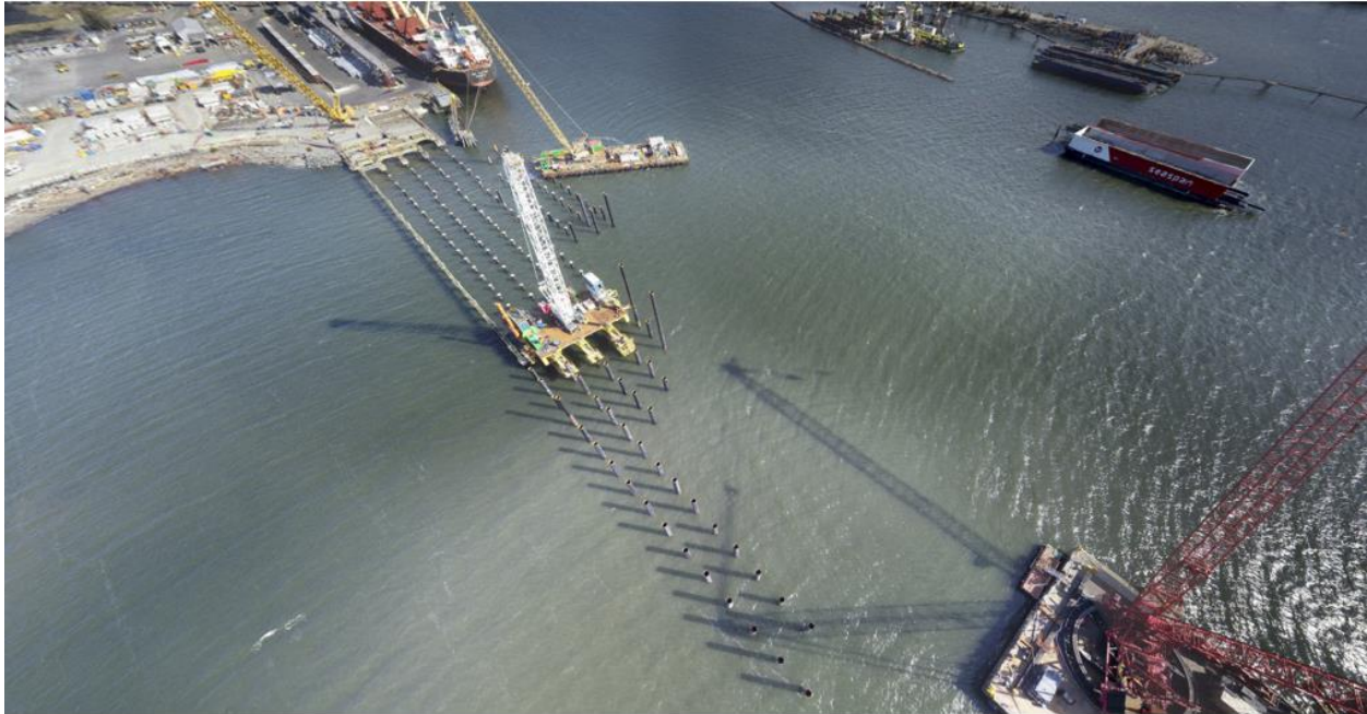
Figure 1 Terminal A construction – piling for foundation
