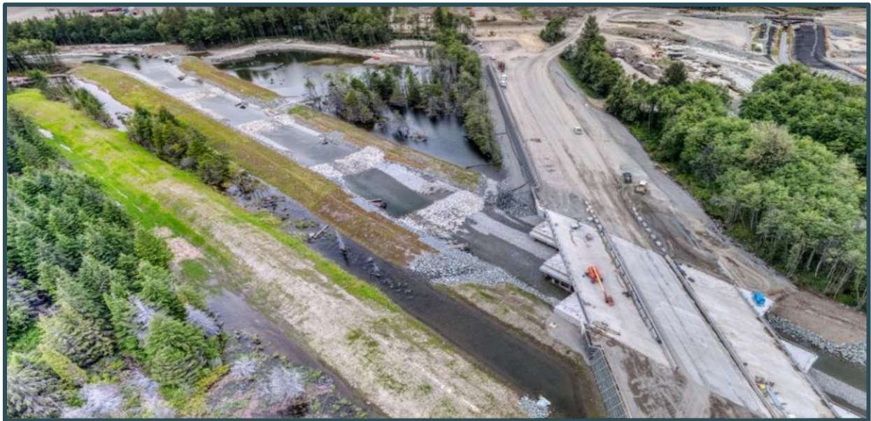
Figure 5 Anderson Creek Diversion and Bridge (Haul Road) AUGUST 2020
