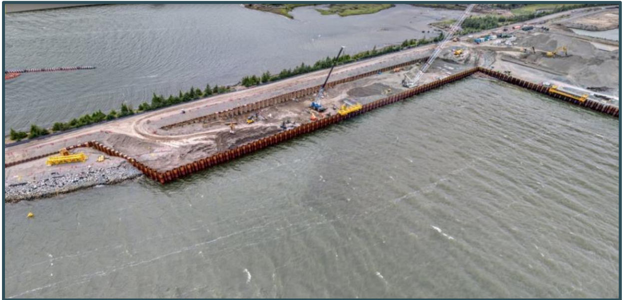
Figure 6 Materials Offloading Facility (AUGUST 2020)
