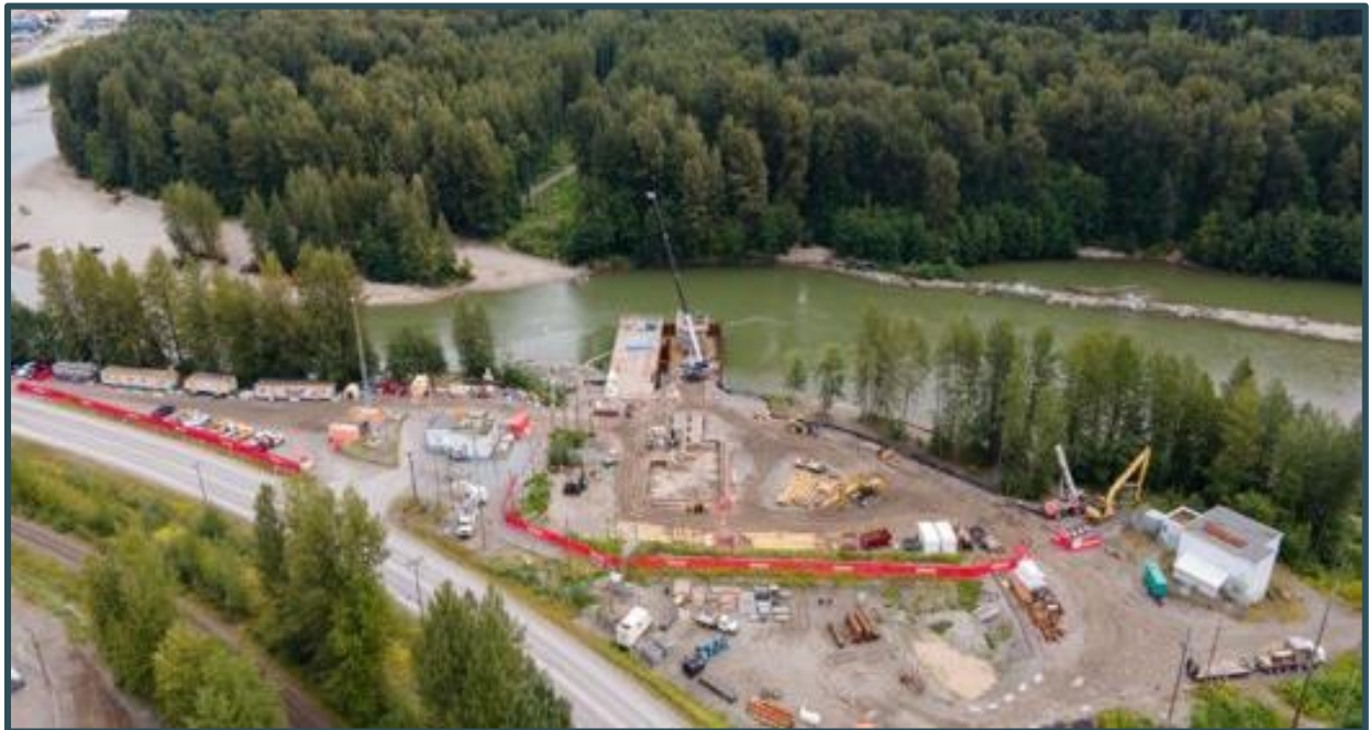
Figure 7 River Water Intake (AUGUST 2020)
