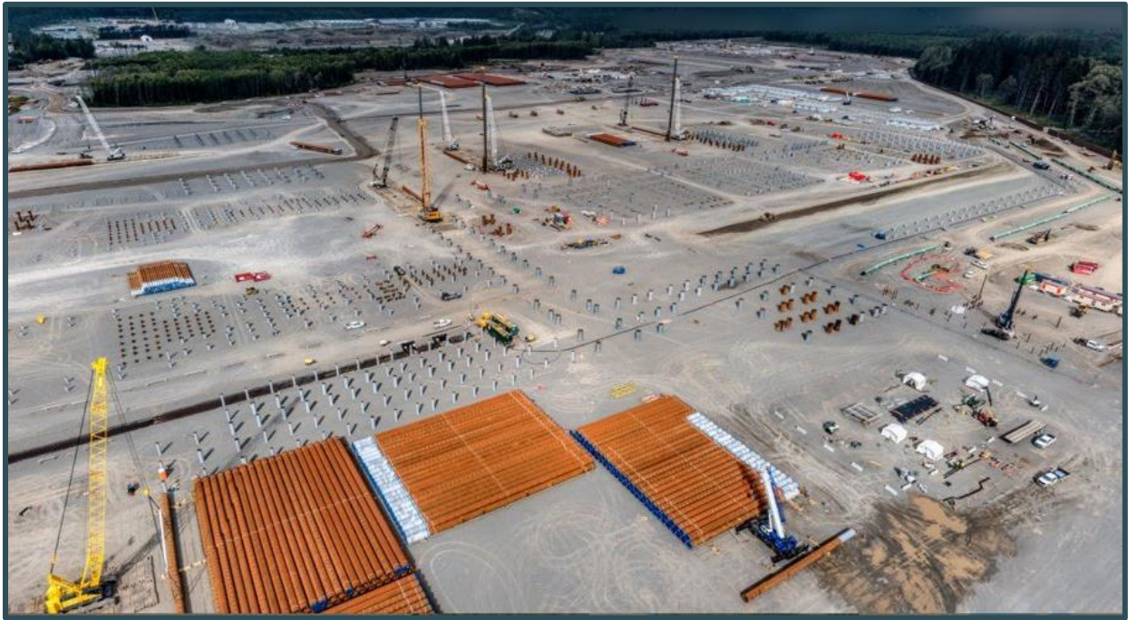
Figure 2 Plant Piling (AUGUST 2020)
