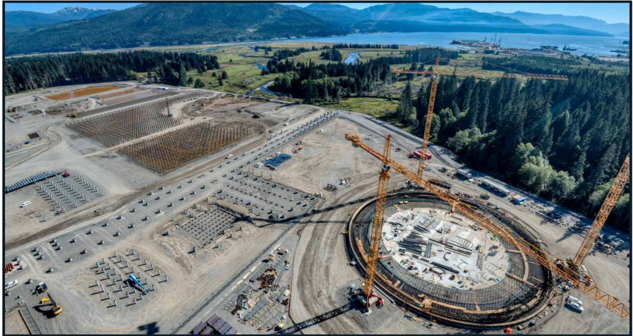
Figure 2 Tank Pad and Piling (September 2020)
