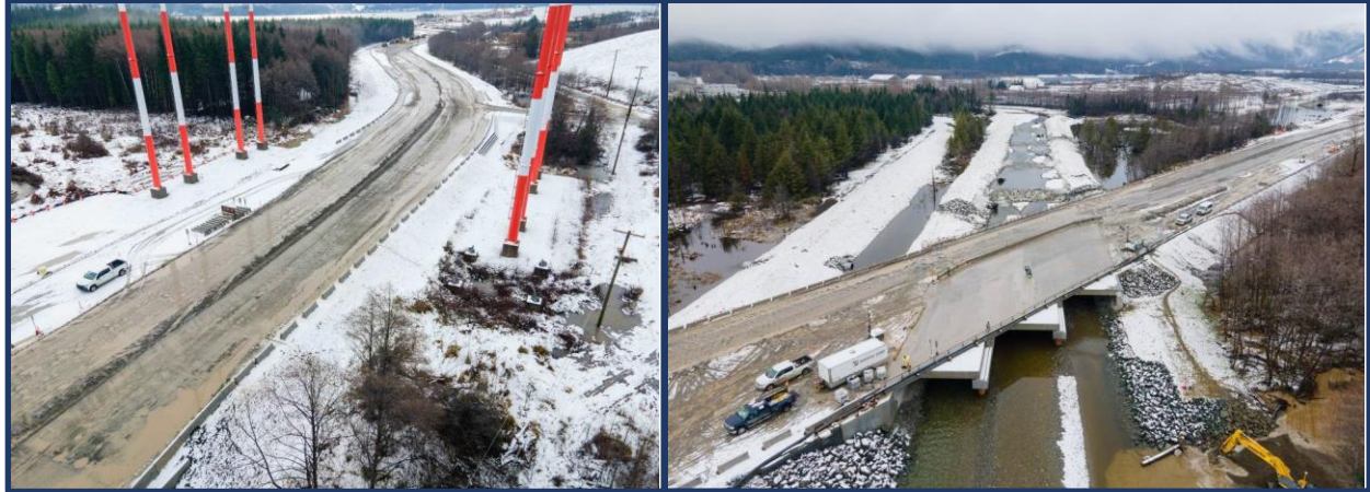
Figure 1 Moore Creek & Anderson Creek Bridges (Q4 2020)
