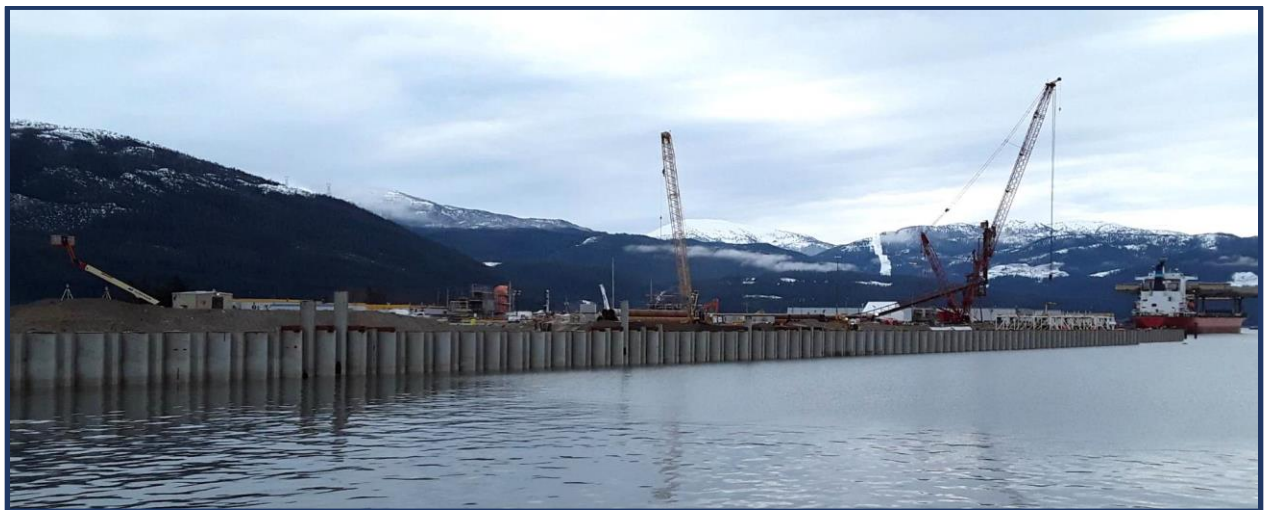
Figure 4 Quay Wall at the Berth (Q4 2020)
