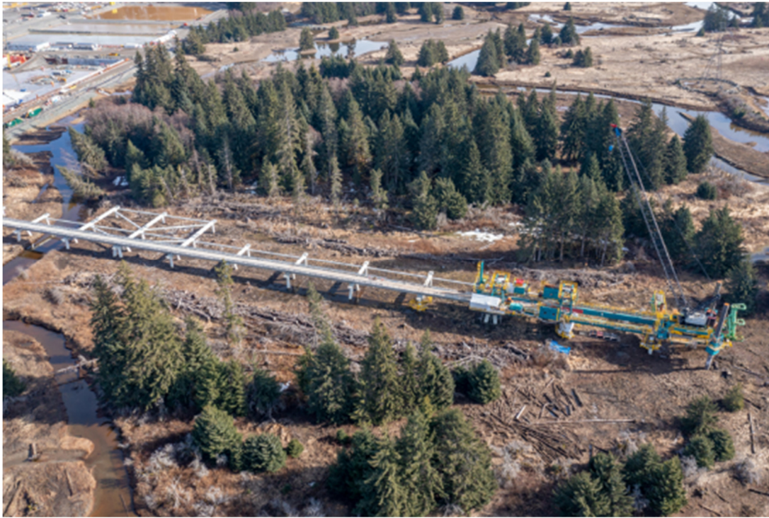
PHOTO 7: CANTILIEVER BRIDGE ON THE LNG LOADING LINE (MARCH 2022)
