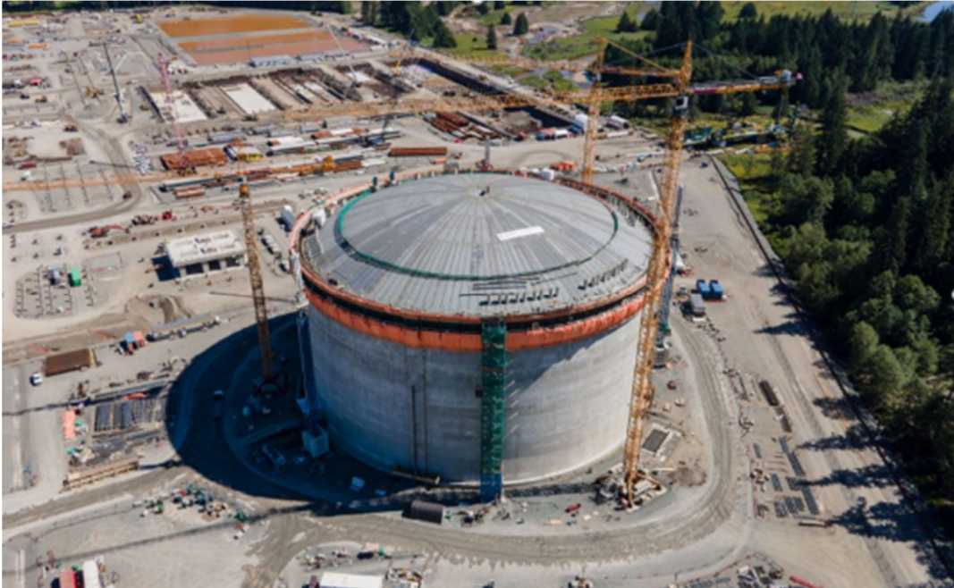
PHOTO 6: COMPLETED LNG STORAGE TANK ROOF RAISE (AUGUST 2021)
