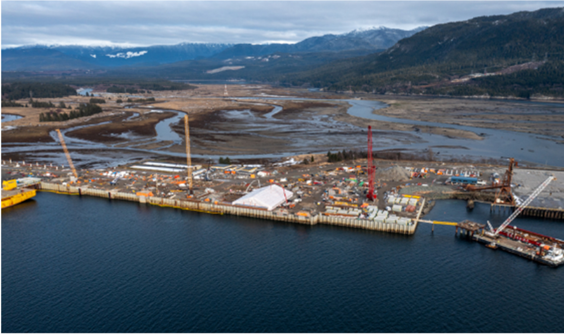
PHOTO 4: BERTH 2 CONSTRUCTION (FEBRUARY 2022)
