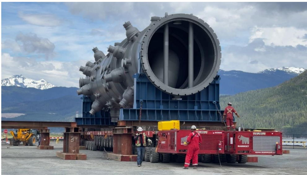
Figure 3.3 Pre-cooler on a self-propelled modular transporter (Q2 2021)
