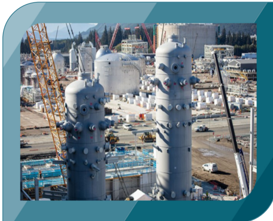
LNG Canada Site Construction Activities, Kitimat, September 2022
