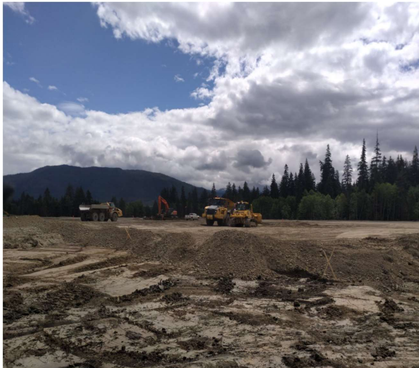
Photo 1 Tank Pad Area
