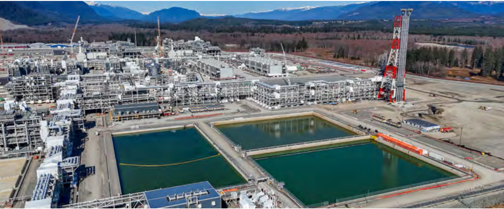
The three ponds at site that hold clean water prior to discharge to Douglas Channel.
