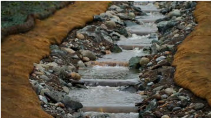
Sumgas Creek fish habitat offset, step pools to support upstream movement of fish.
