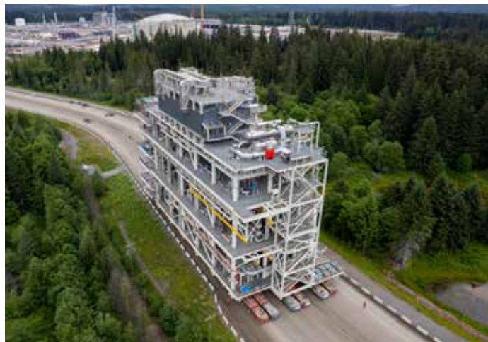
Large module being moved to main operations area
