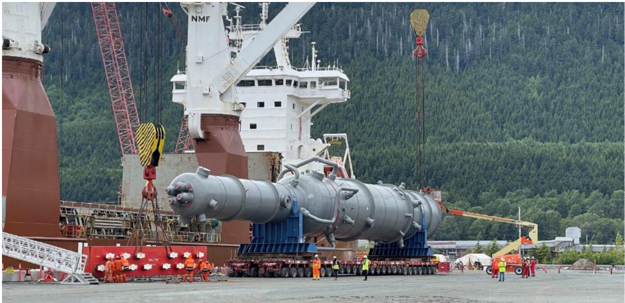
Figure 4 Main Cryogenic Heat Exchanger & Pre-Cooler (2021 Q2)
