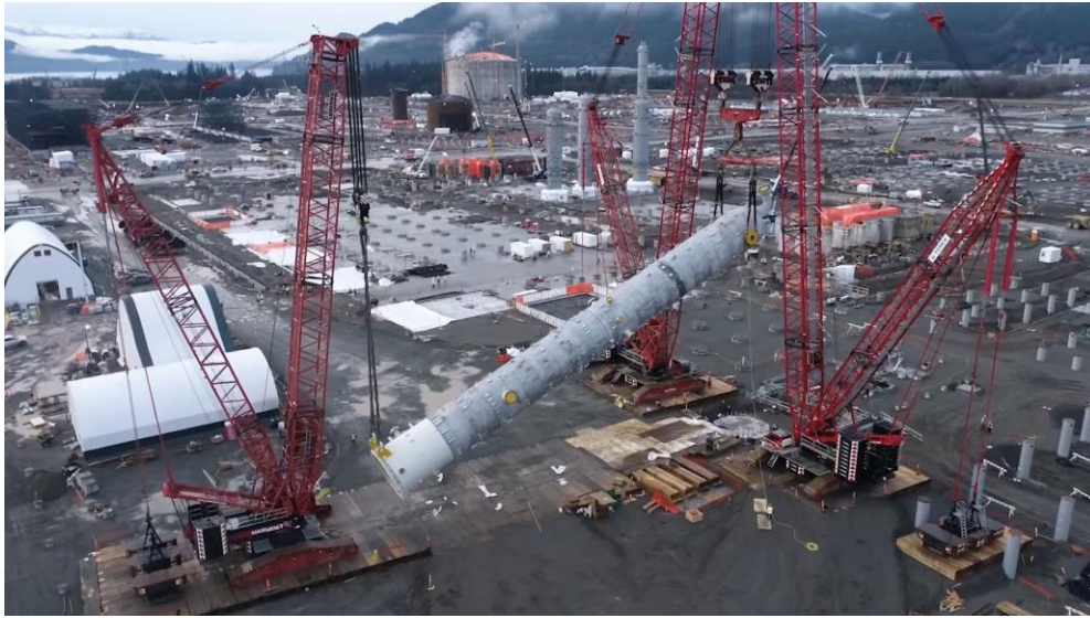
Photo 3 Main Absorber Lift (Q4 2021)
