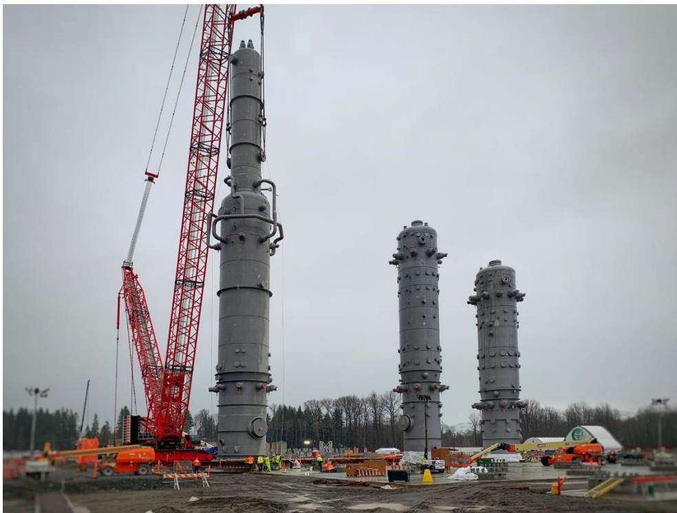
Photo 2 Main Cryogenic Heat Exchanger and two Precooler Units (Q4 2021)
